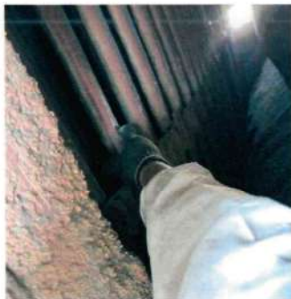
Secondary Supper Heat Tube Thickness Check
